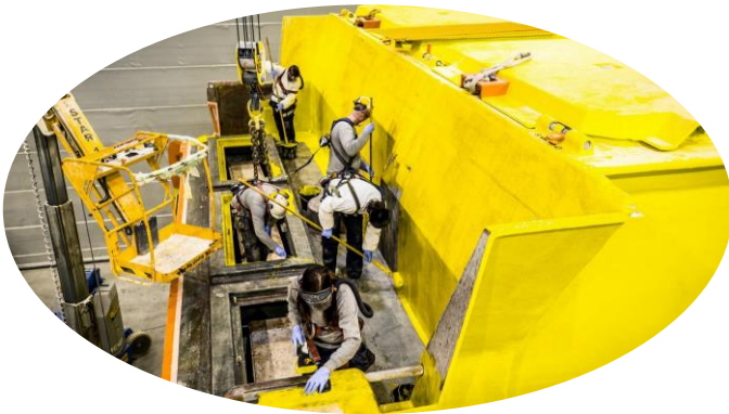
Finishing work (cutting and coating)
