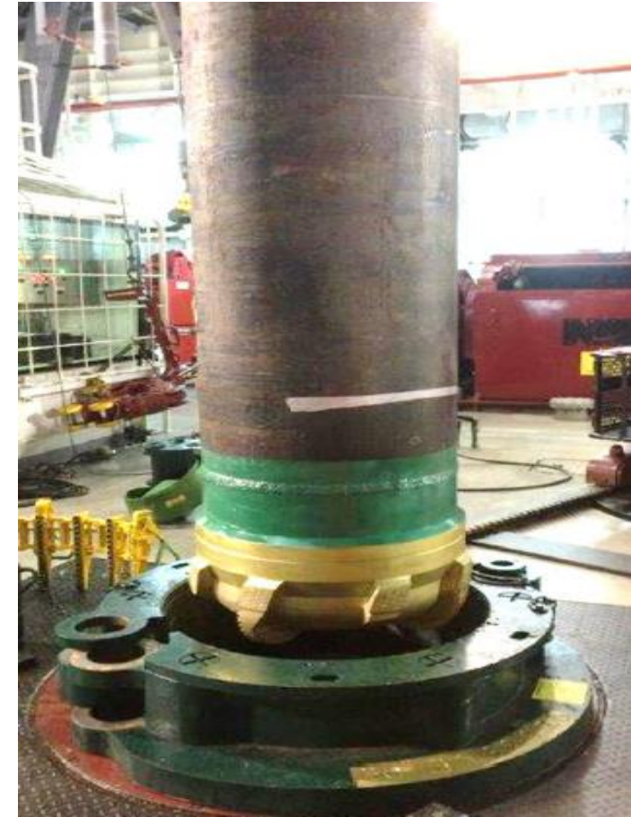
30-in x 34-in. Casing Drilling
